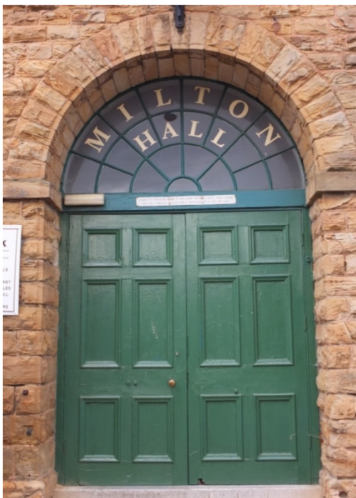
Photos 22 and 23 – 6-panel doors with decorative metal fanlight (Milton Hall) and plain, vertically boarded door with timber fanlight below mock segmental arch (Cobcar Terrace)
