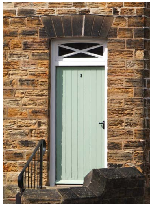
Photos 22 and 23 – 6-panel doors with decorative metal fanlight (Milton Hall) and plain, vertically boarded door with timber fanlight below mock segmental arch (Cobcar Terrace)
