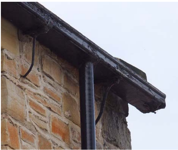
Photo 9 – Wooden box section gutter supported by rise and fall metal spikes
