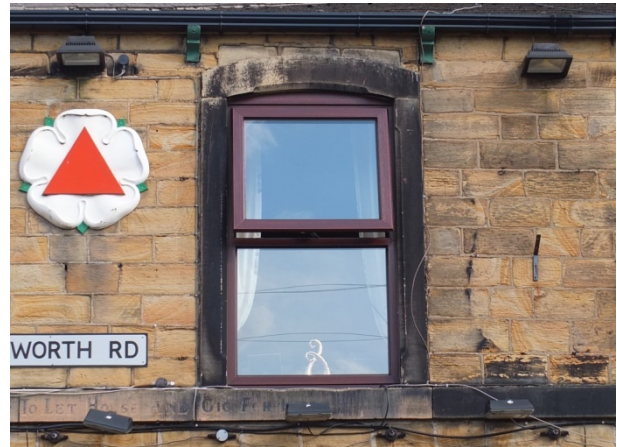
Photo 16 – carved stone head, jambs and sill band to window opening (Market pub)
