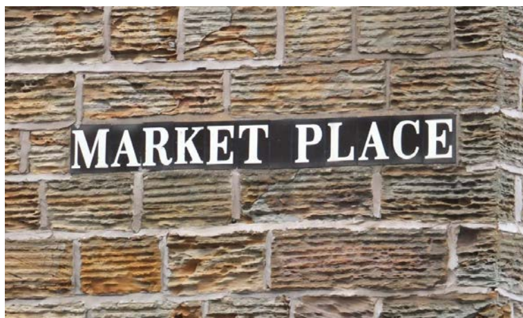
Photo 35 - Inlaid ceramic tile street sign, Market Place, Elsecar
