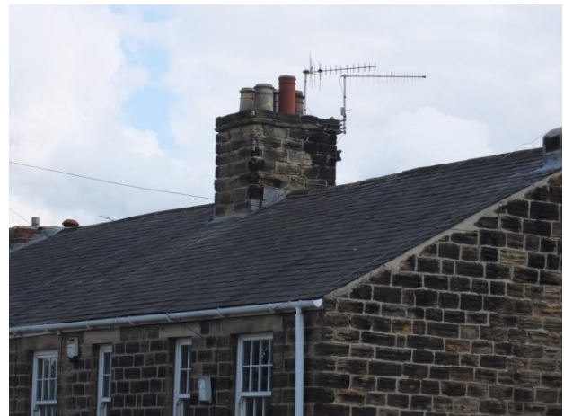
Photo 7 – Welsh slate gable roof with mortar fillet finish
