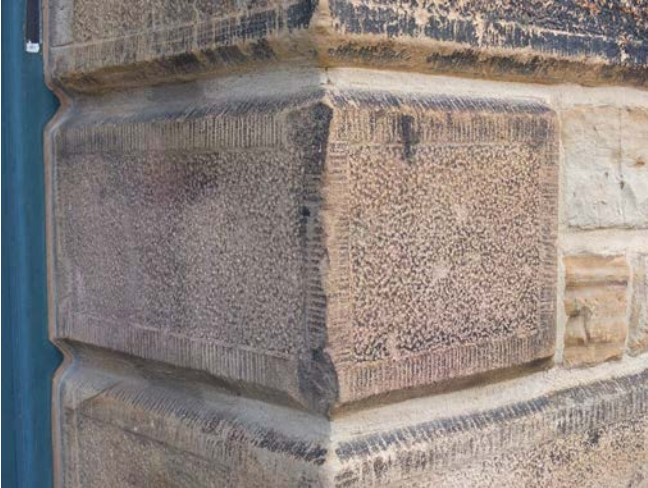
Photo 13 – Pitch faced stonework, in Elsecar this finish tends to be used for quoins (large rectangular stones at the corners of walls)
