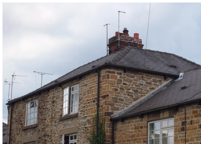
Photo 5 – hipped Welsh slate roof (Station Row)
