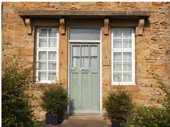
Photo 17 – simple stone canopy with stone corbels (Fitzwilliam Street)
