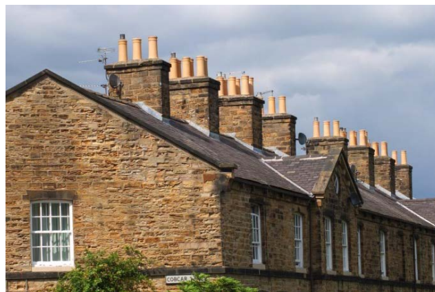
Photo 3 – restored chimney pots, Cobcar Terrace
