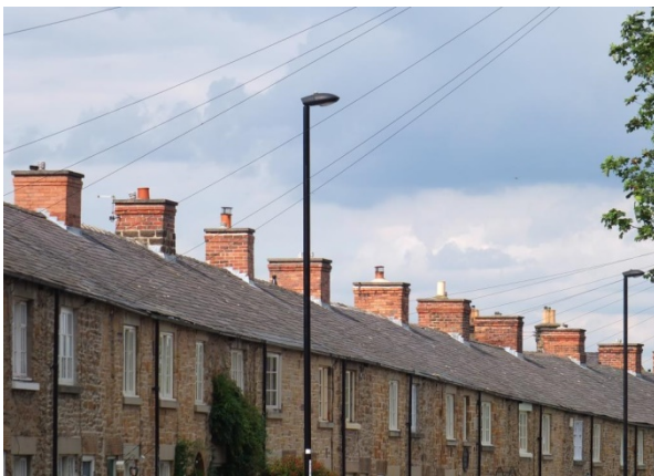
Photo 1 – replaced brick flues on Reform Row with simple high level string course
