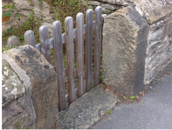
Photo 30 – Gate posts with simple carved tops and gate set behind
