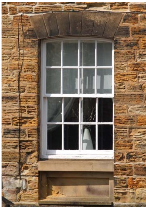
Photos 24 and 25 – timber sliding sash windows of different types, with narrow glazing bars
