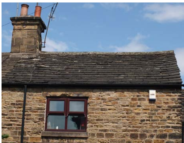
Photo 4 – stone flag gable roof (Fitzwilliam Street)
