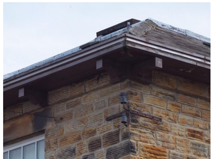
Photo 10 – Wooden box section gutter supported by wooden corbels
