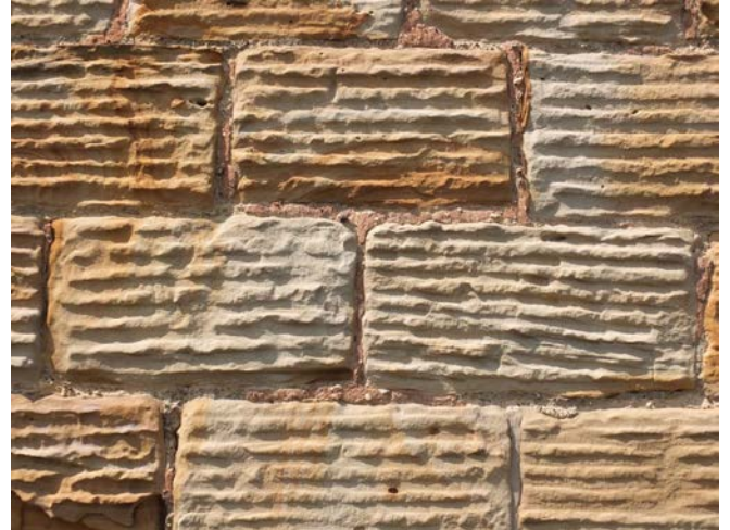
Photo 14 – Parallel punch stonework, a common design feature seen in Elsecar on the exterior of historic buildings
