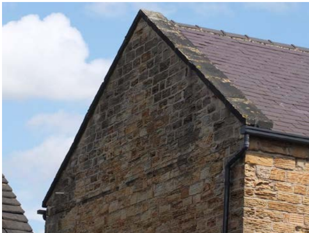
Photo 6 – Welsh slate gable roof with verge coping
