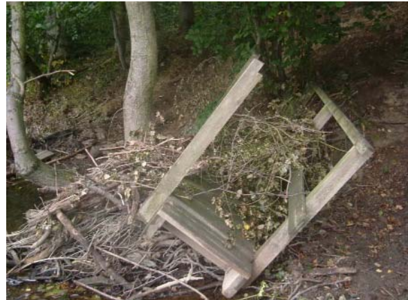
Bridge over (or not) Rons Cliff Dyke
