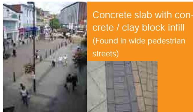
Concrete slab with concrete / clay block infill (Found in wide pedestrian streets)
