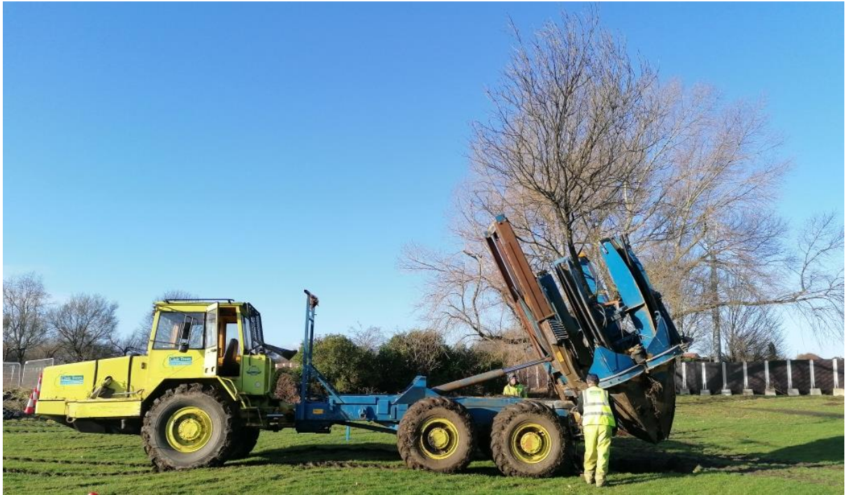
Above: Tree being relocated.
