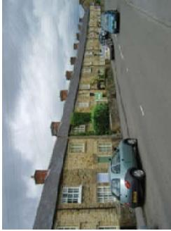
Figure 29:The pattern of the new repair and original finish to stonework and windows is evident on Reform Row
