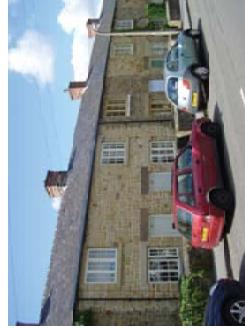
Figure 30:Heavily eroded stonework on the southern corner of Reform Row. Repairs to mortar actually stand proud of the missing faces of the blocks, testament to 170 years of exposure
