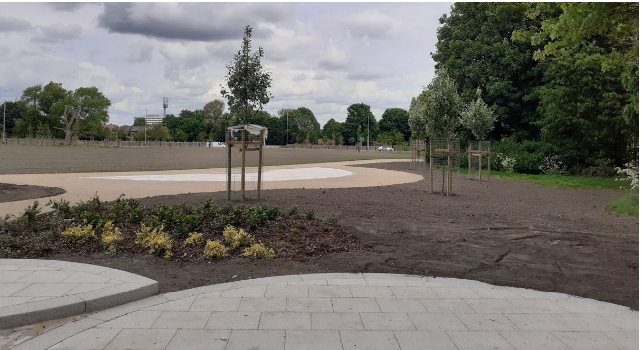
Above: Flexipave footpath towards main entrance, patio and planted area in front of the newly clad community cabin.
