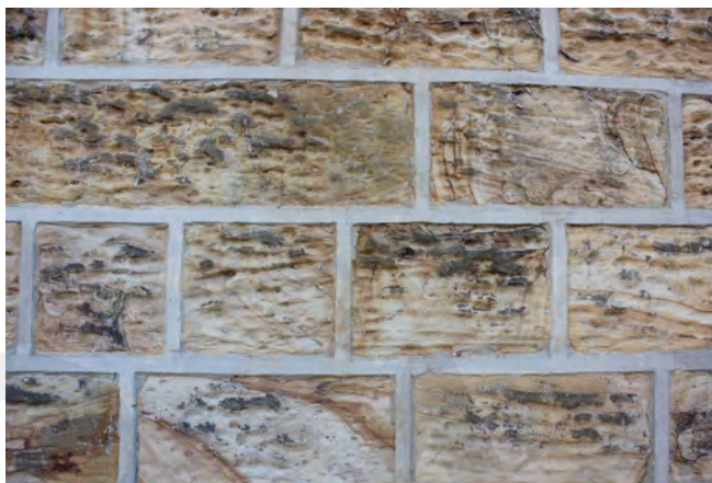
Strap pointing is not traditional and is inappropriate within the Conservation Area. Additionally, the use of cement mortar will cause further decay to the already weathered stonework
