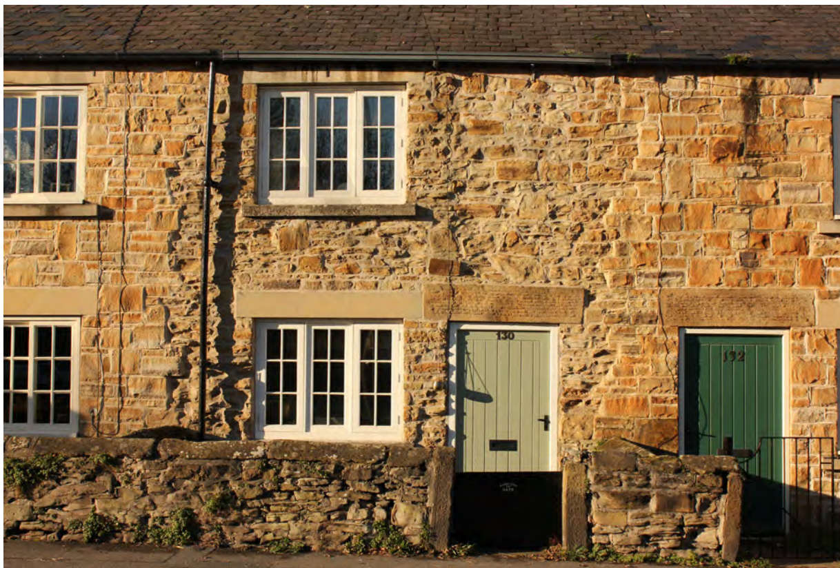
Different repair methodologies and on Reform Row have impacted on the uniformity of the façade
