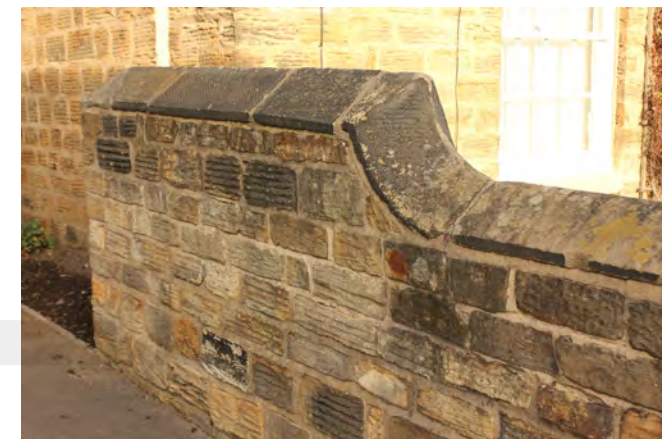
Traditional boundary wall with chamfered coping
