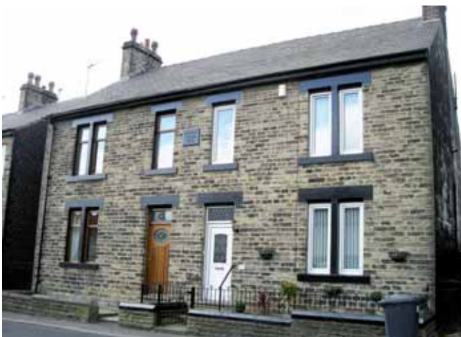
The low wall and small set-back in Dodworth, Barnsley provide an effective transition while maintaining enclosure
