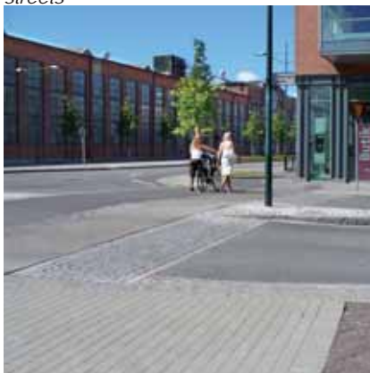
A speed reduction strategy could include raised crossings and small kerb radii
