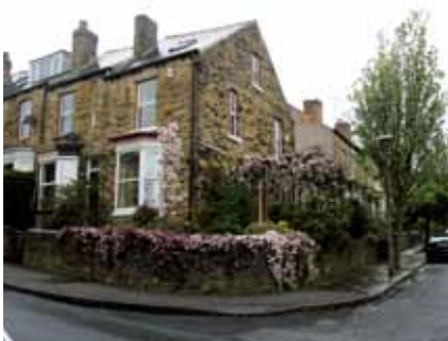
This end terrace in Crookes, Sheffield turns the corner with a door and windows on the gable end
