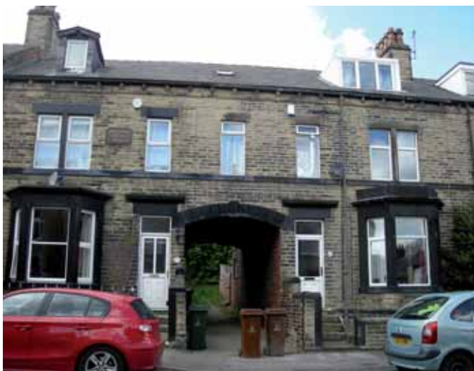
The traditional 'ginnel' is a robust and adaptable feature that allows for access to waste and recycling storage that remains out of view
