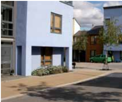
A shared space street with areas identified for pedestrians (other features may be necessary in some situations to define the protected zone)
