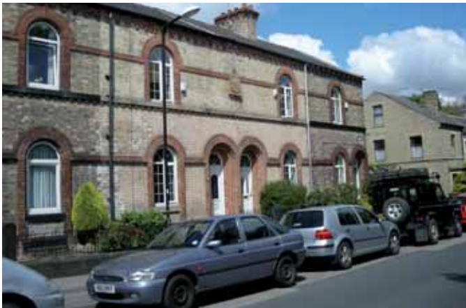
The combination of active openings and more elaborate detail in Old Town, Barnsley, create a strong public front to the building
