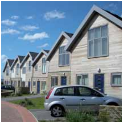
Front off-street parking is convenient but can dominate a street if not broken up
