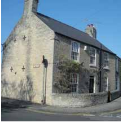
Double pitched roofs with gable ends like this one in Tickhill, Doncaster, are one of the predominant roof forms in South Yorkshire
