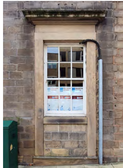
Altered door and intrusive cable trunking
