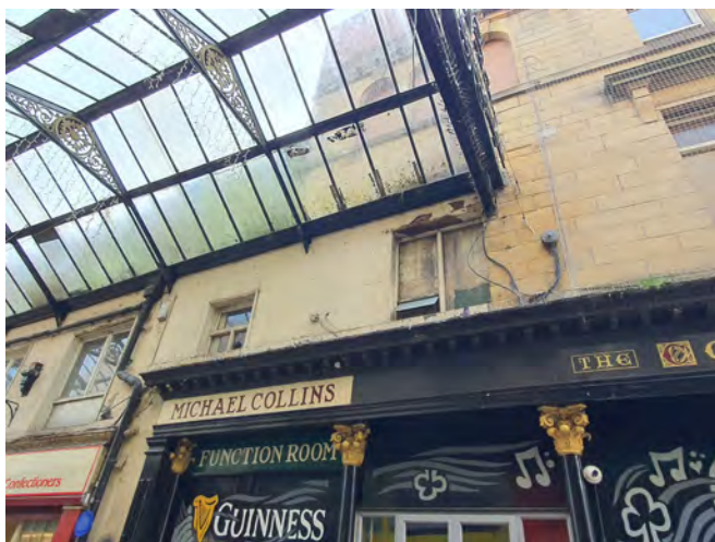
Guano accumulation, bird netting, bird spikes and poor maintained upper storey in the arcade
