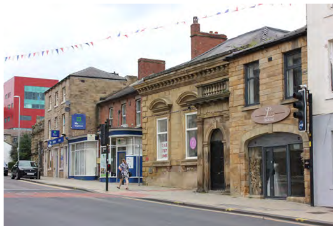
A variety of buildings feature in the character area; Barnsley College looms in the background
