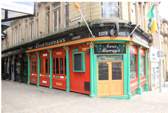
Cast-iron Corinthian columns on this former shop front on Market Hill
