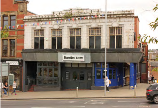
Interesting 1930s building on Shambles Street
