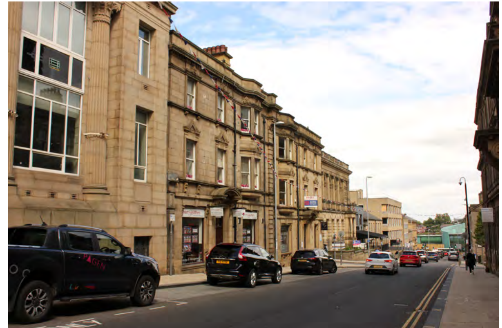
Busy traffic on Regent Street along with on-street car parking bays
