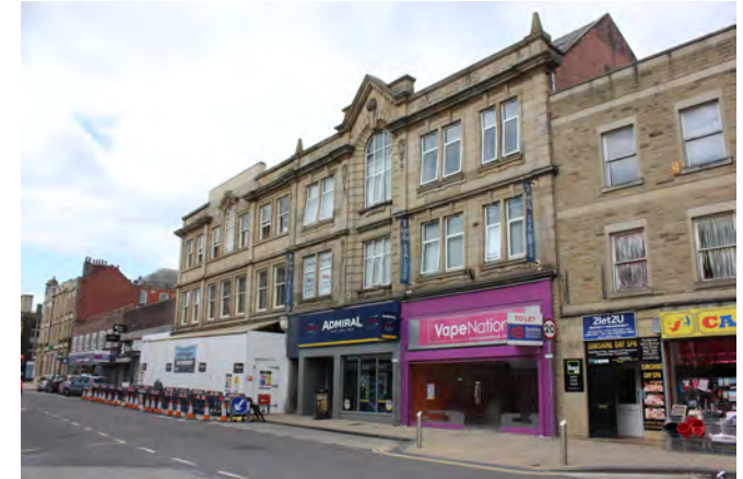
Former YMCA and Eldon Buildings
