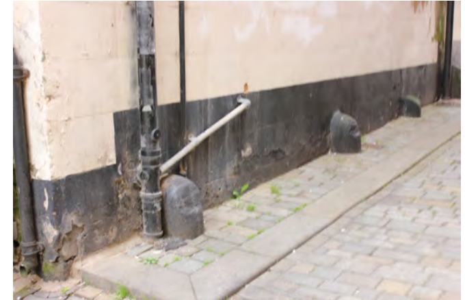
Spur stones at the entrance to George Yard from Market Hill
