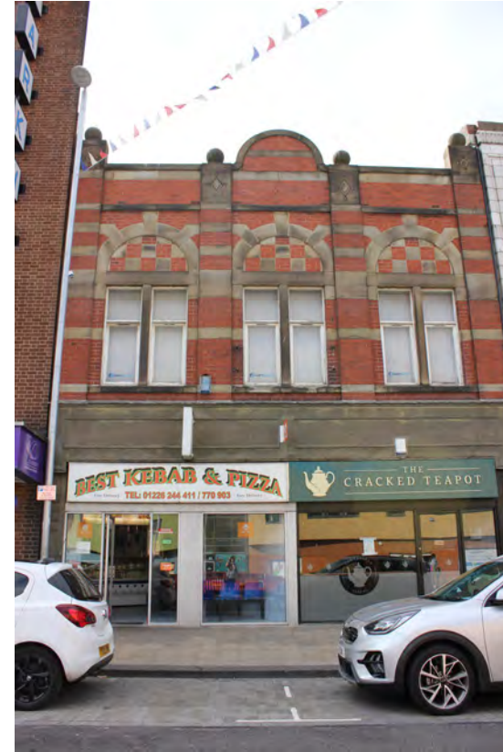
Unusual red brick at No.70 and 72
