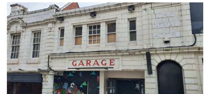
Detail of the Royal Street Garage
