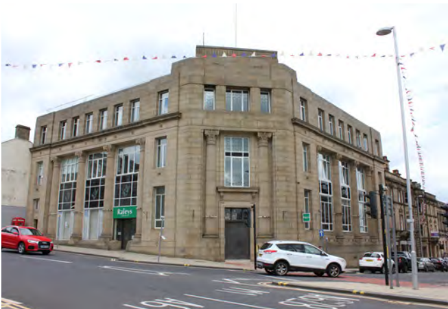
The Permanent Building, corner of Church Street and Regent Street
