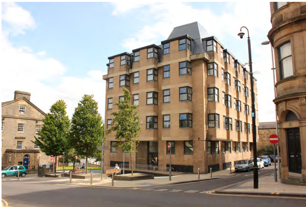
Converted offices on Regent Street
