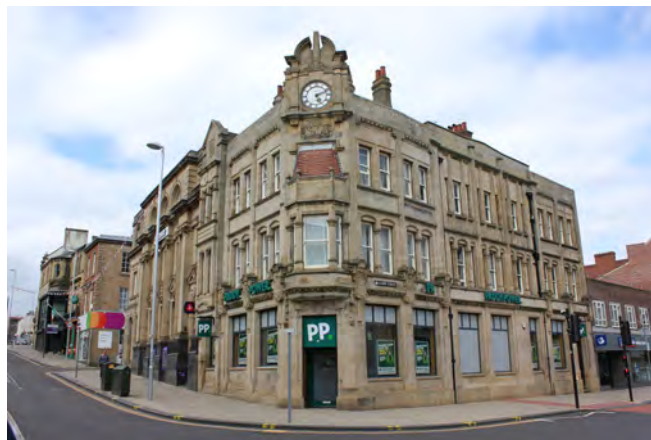
Former Yorkshire Penny Bank, corner of Market Hill and Eldon Street and Grade II listed
