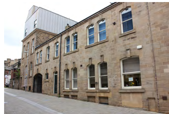
The rear elevation of Queen's Court, the former Queen's Hotel, with overly large roof extension
