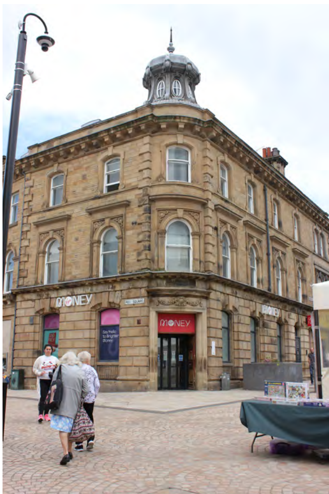
Former Yorkshire Bank, built as the Coach and Horses in 1857 with lead dome added in 1912
