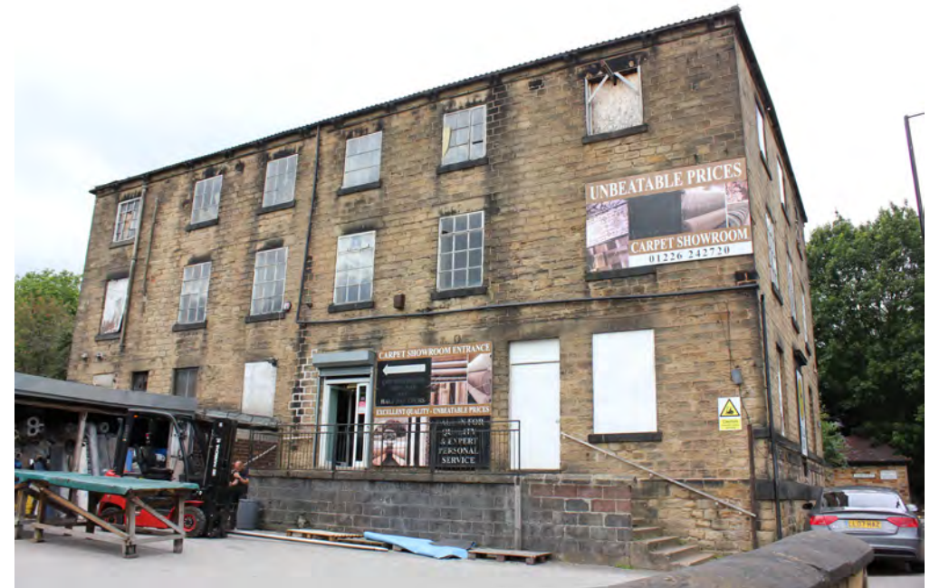
Cass's Warehouse a former linen warehouse
