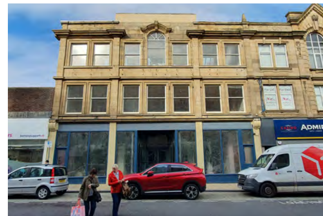
The former YMCA on Eldon Street once had distinctive shopfronts with curved glass – this traditional shopfront replaces a less-than sympathetic shopfront as part of the HAZ.
