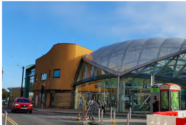
Interchange combines a bustling bus and rail station on the edge of the conservation area
