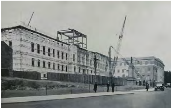
The Town Hall under construction.
