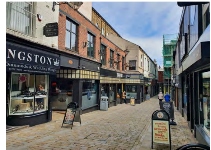
Eastern end of the Arcade
