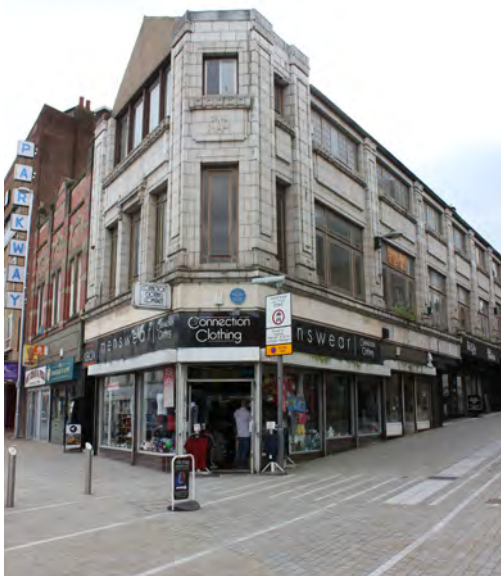
Nos.2-10 Eldon Street with faience façade
